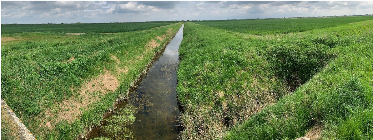
Photos 3 and 4: Field Ditches and Bridges
