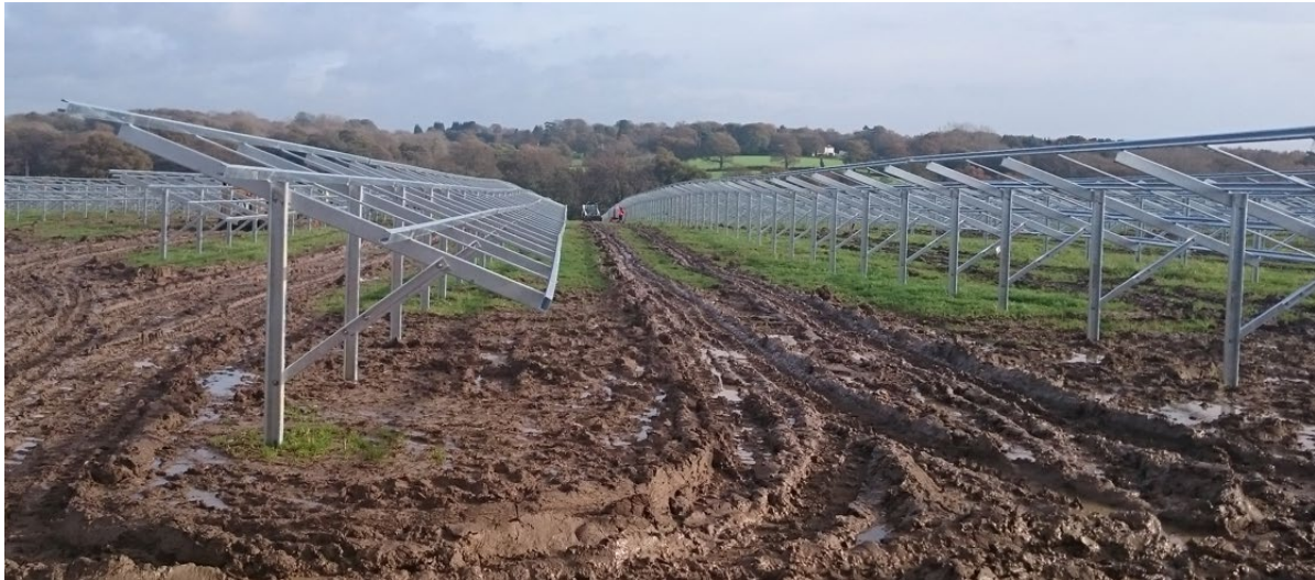
Photos 20 and 21: Restoration of Light Surface Damage
